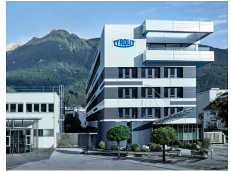
Tyrolit headquarters in Schwaz (Austria)
