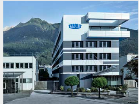
Tyrolit headquarters in Schwaz (Austria)
