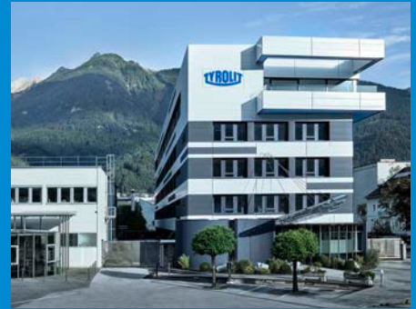
TYROLIT headquarters in Schwaz (Austria)
