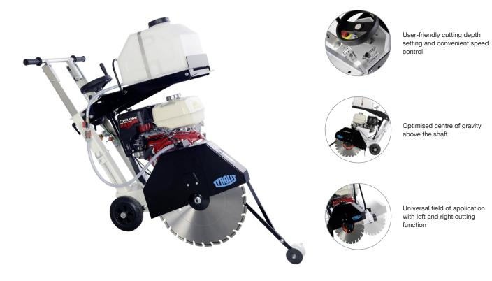
Thanks to its extremely robust, high-quality chassis, the FSG513 is highly robust and flexible thanks to the left- and right-handed as well as corner flush cutting functions. The reliable Honda petrol engine is equipped with a cyclone air filter.
